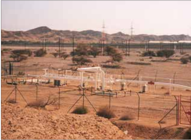
GAS PIPELINE FENCE AND GATE
