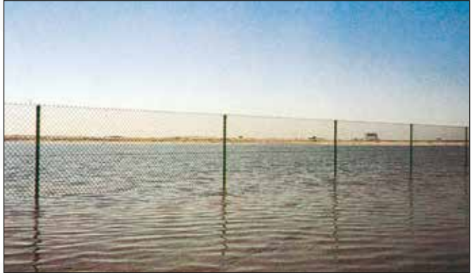
PVC COATED FENCE INSTALLED IN SEAWATER
